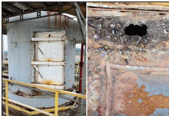
Bag house structure with corroded breach.
