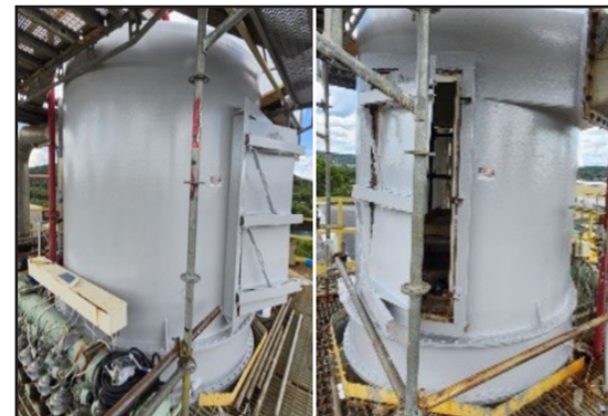
ARC CS2 applied as top coat over CFW-CR repairs.
