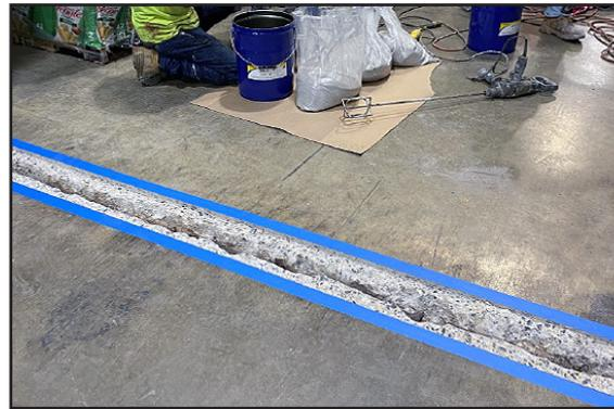
Damaged joint prepared for repairs with EG-1 FC patch kits.
