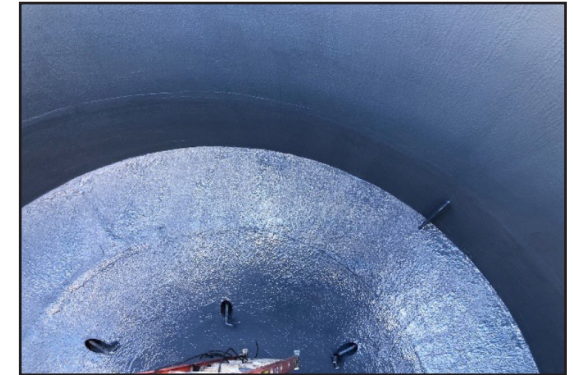
Second of two coats of ARC SD4i after application.
