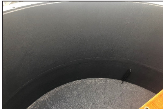
Blasted surfaces being repaired with ARC 858.
