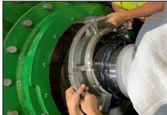
The 442 Split Seal was adapted to fit the stuffing box.
